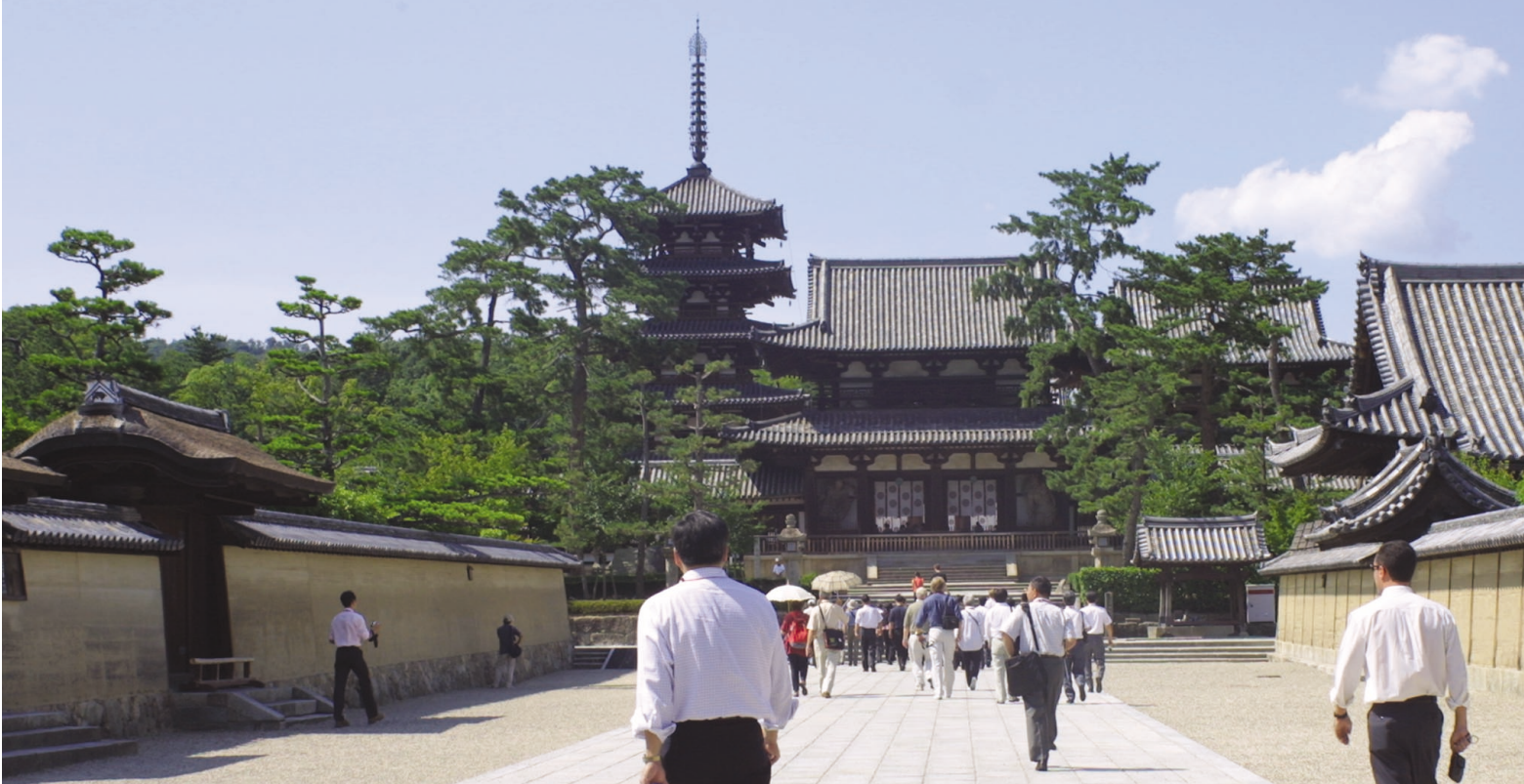
The IMLB-12 conference included an excursion to Horyuji Temple, the world's oldest wooden structure, located south of Nara.
