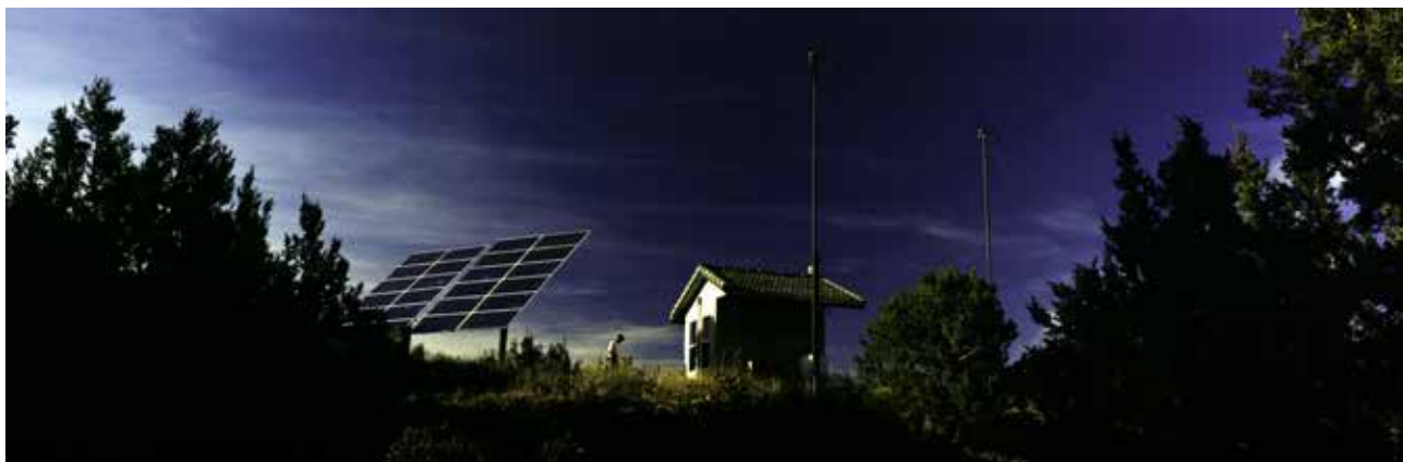
Fig. 1. Remote PV, wind, and battery storage system for a Colorado residence. (Photo by Warren Gretz, NREL 10622.)
