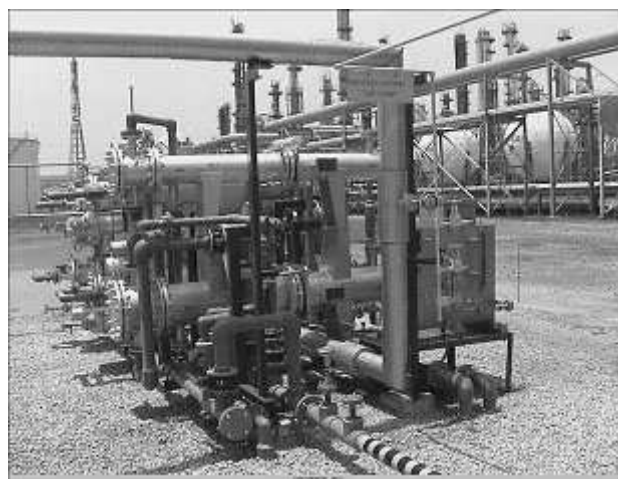
Fig. 2: Mock – up heat exchanger located inside a petrochemical plant on Jurong Island.
