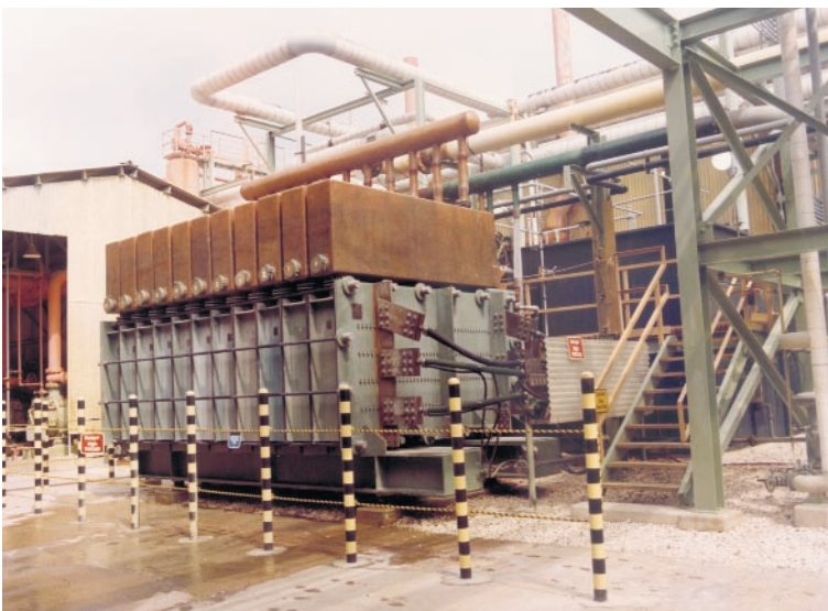
FIG. 4. Assembled Glanor V-1144 Electrolyzer at Lake Charles "Plant C."
